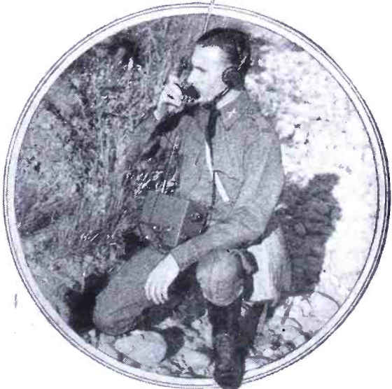
↑ Weighing only 10 lbs., U.S. Army "transceiver" has reliable range of 4 miles ↓
