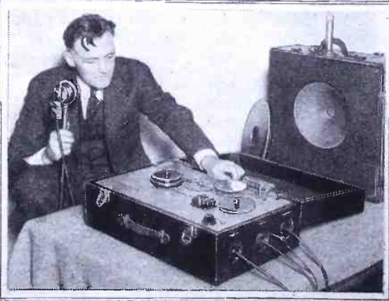
Recording sounds on endless steel tape 81 ins. long and 0.0015-in. thick, shown at right. It will play back the sounds instantly like an echo. A signal light warns when to stop talking.
