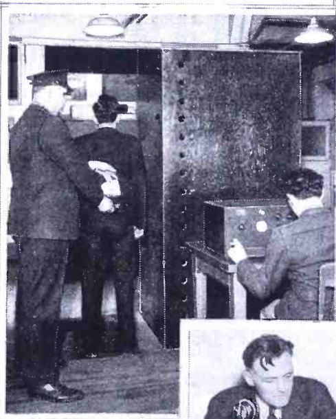
Recording sounds on endless steel tape 81 ins. long and 0.0015-in. thick, shown at right. It will play back the sounds instantly like an echo. A signal light warns when to stop talking.
